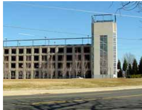
A windowed stair tower prominently occupies the corner of this parking garage, making it easy to both find the entry/exit and be seen inside.
