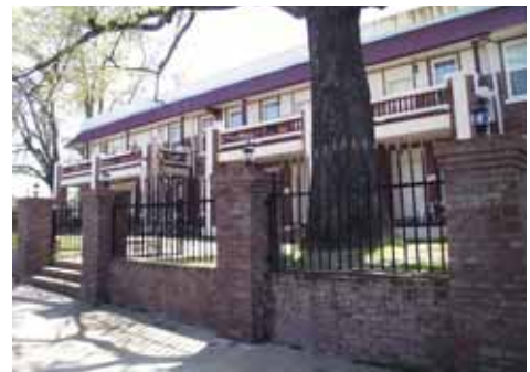
Decorative metal fencing is combined with a low brick wall and piers to create an attractive street edge.
