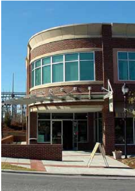
Traditional facade details such as cornices, canopies, and recessed storefront entries, are reinterpreted in the design of this modern building.
