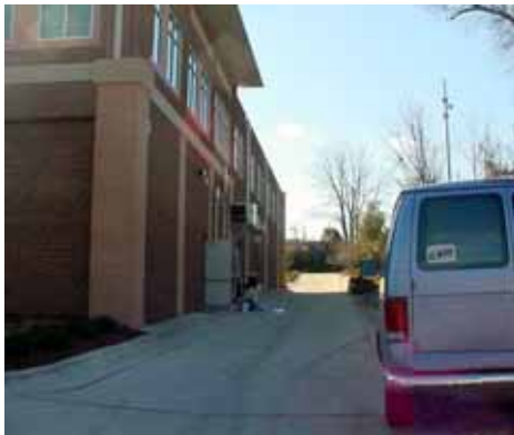
A rear service alley provides deliver access and hides utility boxes and meters.
