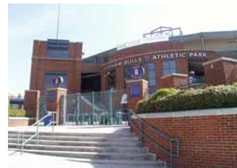
A contemporary ballpark uses traditional brick to reinforce the pedestrian scale, provide a low maintenance facade, and maintain continuity with historic tobacco warehouses across the street.
