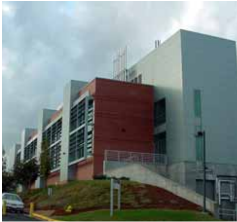
The varied roofline conceals rooftop equipment from view and helps to reduce the bulk of the building.
