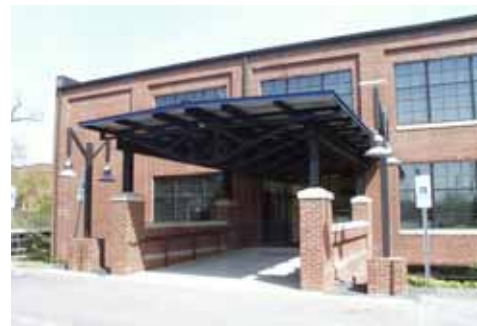
A generous covered entry is both functional and easily recognizable. Lighting on either side of the entry further emphasizes the portal at night.
