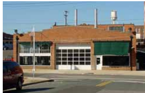
A former garage leads a new life housing the offices and labs of a biotechnology
