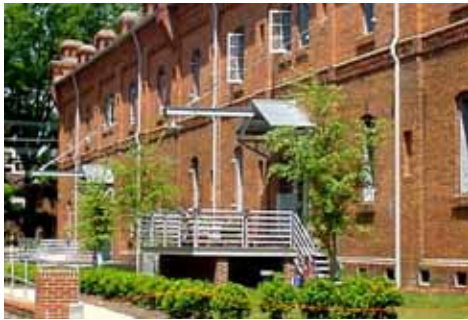
A residential adaptive reuse complex unites a variety of brick tobacco warehouses with consistent metal railing and canopy elements.
