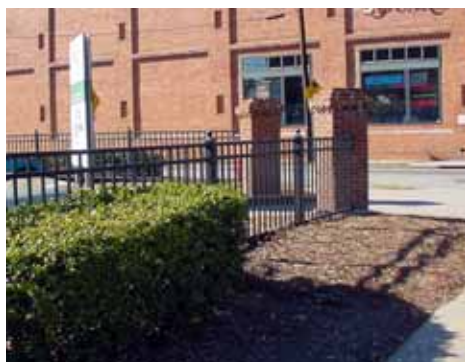
Brick piers mark the opening in the decorative metal fence and relate it to the surrounding architecture. Landscaping on the street side of the fence adds variety and color.
