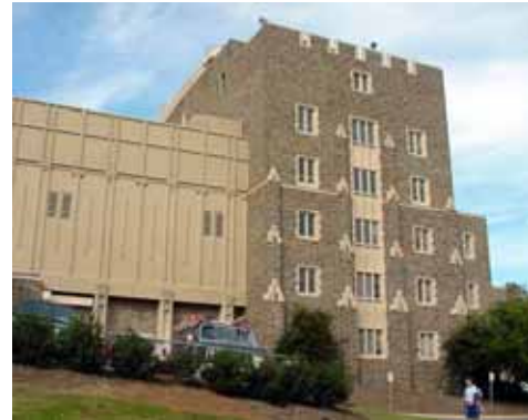
A massive wall's scale is reduced through changes in material. A monolithic concrete wall is detailed with insets to give relief to an otherwise blank wall.
