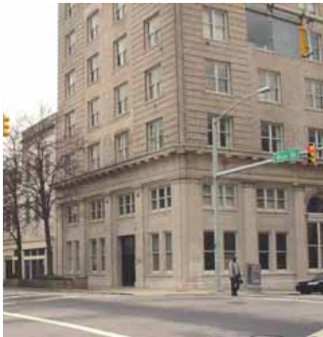
The lower, street level stories are differentiated from the upper stories by materials, finishes, and the level of detail.
